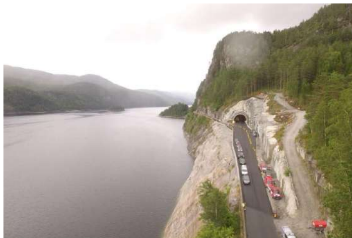
Figure 10 - Bjørkås tunnel bypassing hazardous rock fall areas along the coast
