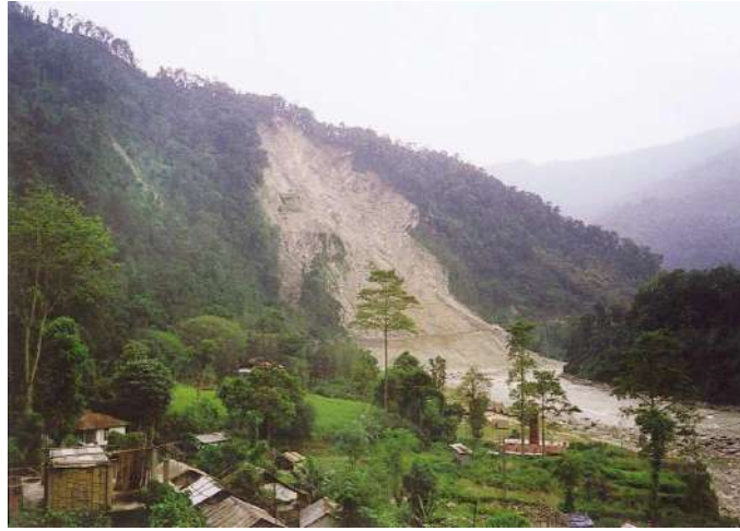
Figure 7a - The Burdang slide on National Highway 10
