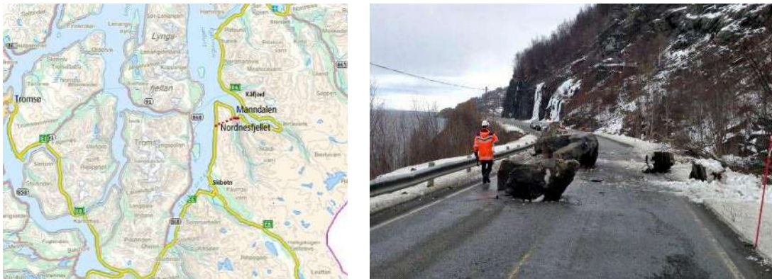
Figure 12 - Rock fall on the road in Nordnesfjellet (North Norway near Tromsø)
