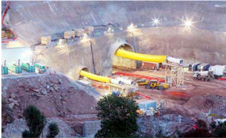
Figure 2 - A view of Chenani-Nashri main and escape tunnels (Photo: dailyexcelsior.com)
