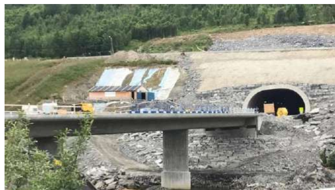
Figure 13 - The entrance to Nordnes tunnel from the Mandalen side
