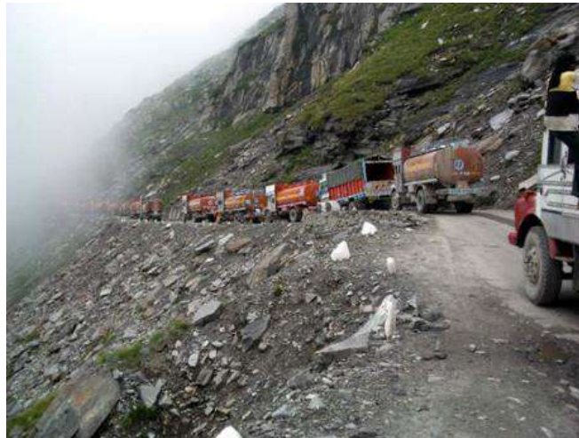
Figure 3b - The original road above the Rohtang pass (John Hill, 2007)
