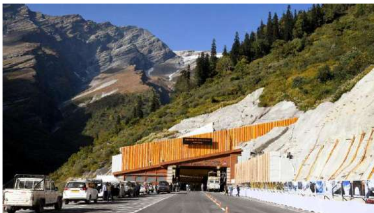
Figure 3a - The southern portal at Rohtang pass
