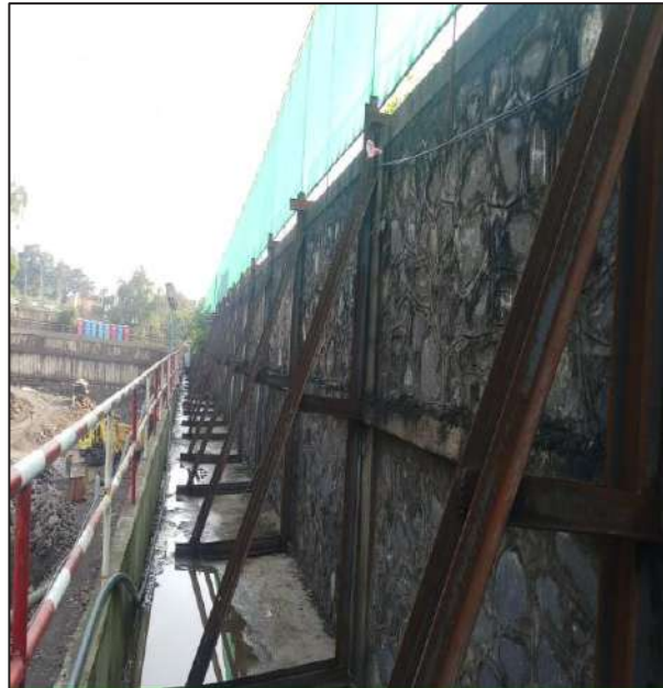
Figure 10 - Hutment wall protected by Shoring at civil court station
