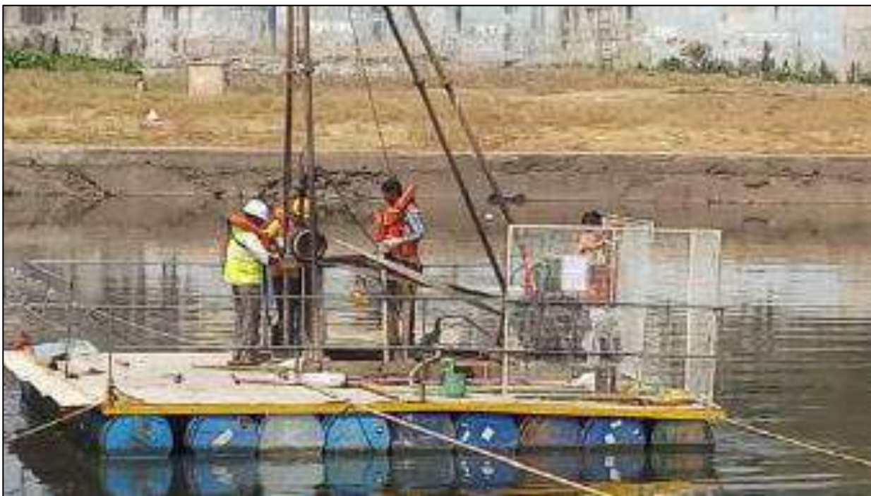
Figure 16 - showing the geotechnical investigation work at tunnel alignment.
