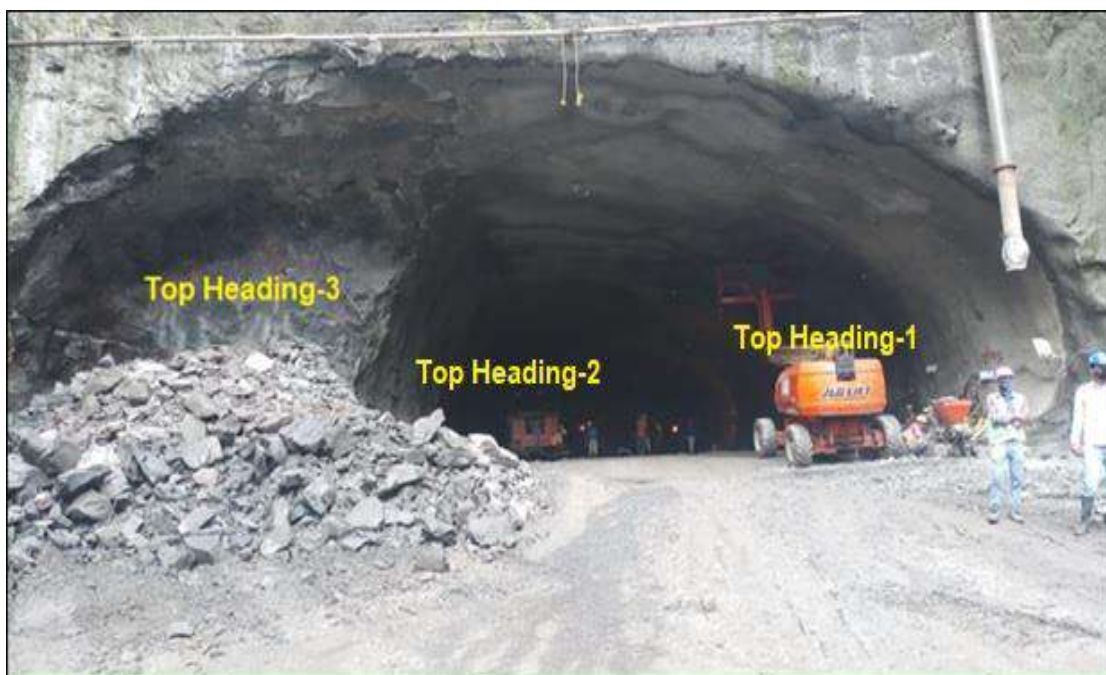
Figure 7 – Excavation using NATM in cross over tunnel at Swargate station
