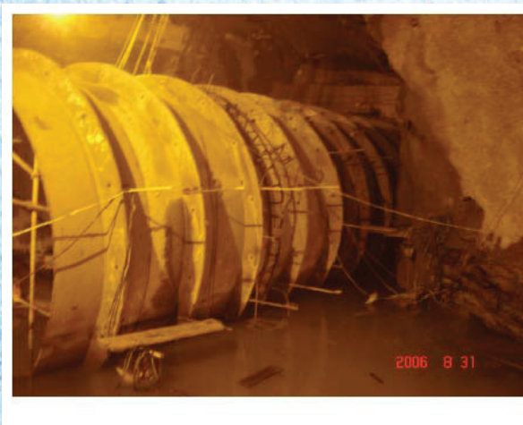
Fig 3: Steel Liners for Penstocks with Stiffeners
