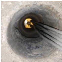
Fig. 10 - Installation of anchors and extensometers
