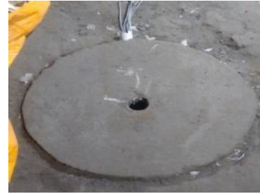
Fig. 9 - Concrete pad for plate jacking test
