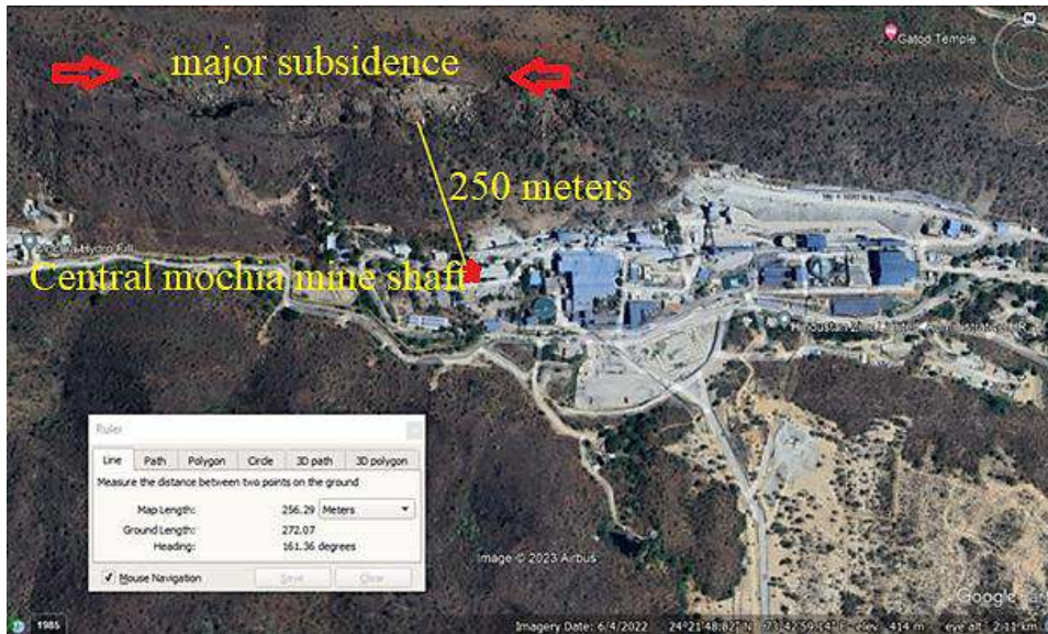
Figure 2 - Areal view of Central Mochia mine shaft indicating major subsidence
