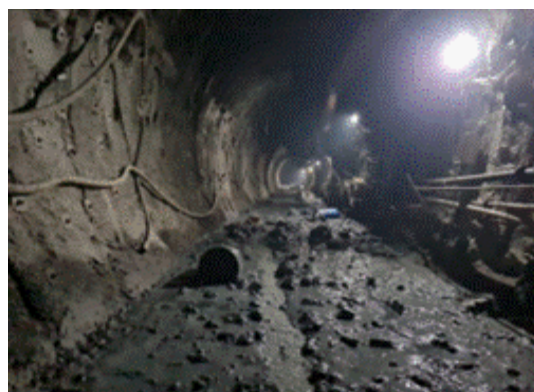
Figure 3b - Mud flow deposit after the 1 st collapse
