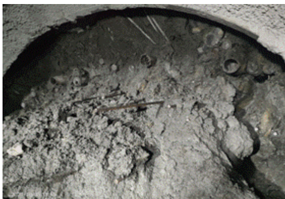
Figure 3a - Tunnel face bulged before the collapse
