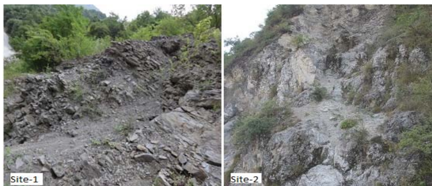
Figure 2 - Field photographs showing weathered rock mass observed at sites
