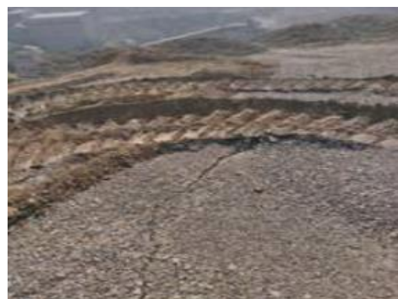
Fig. 2 - Tension cracks present on the dump
