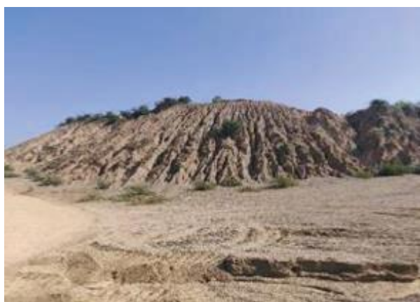
Fig. 1 - Traces of erosion on dump slopes
