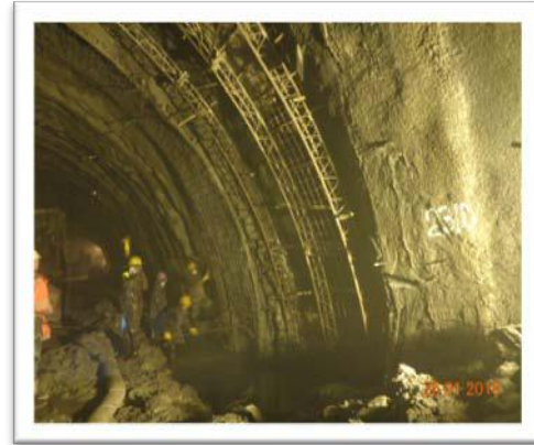
Figure 27 - Re-profiling and lattice girder support
