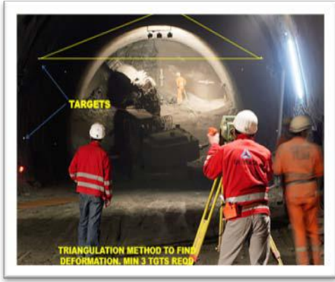
Figure 26 - 3D deformation monitoring
