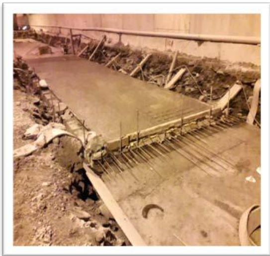
Figure 37 - Concreting of base slab
