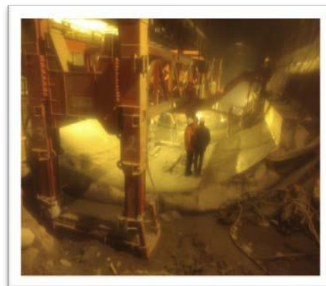
Figure 34 - Lining of deep invert
