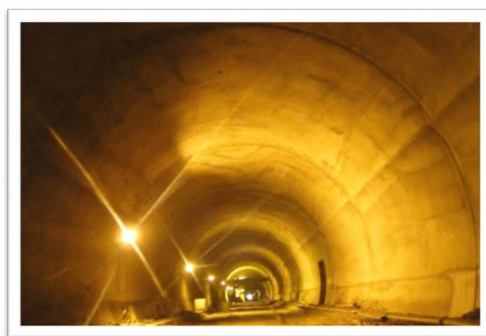
Figure 41 - Completed final lining of overt
