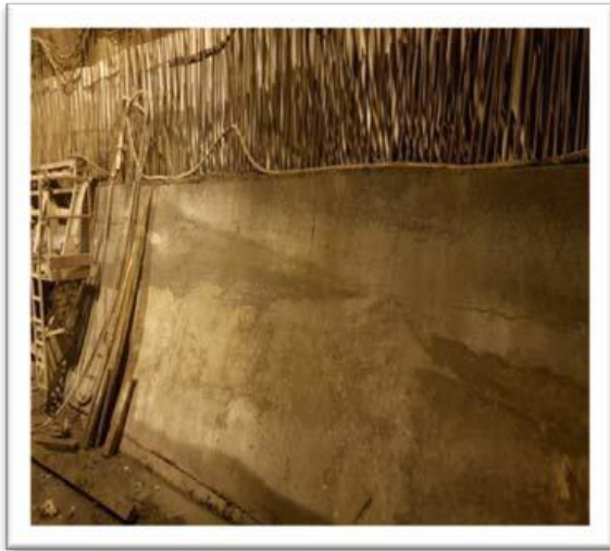
Figure 35 - Reinforced kicker lining
