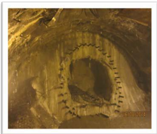
Figure 22 - Pilot tunnel
