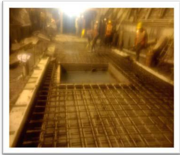
Figure 36 - Reinforcement of base slab
