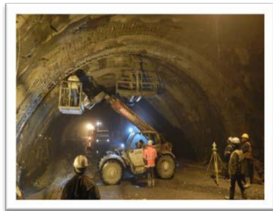
Figure 25 - Saw tooth filling
