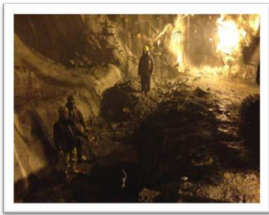
Figure 24 - Excavation for temporary invert
