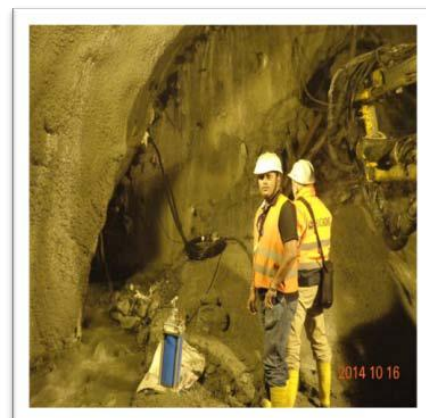
Figure 16 -Water pressure test
