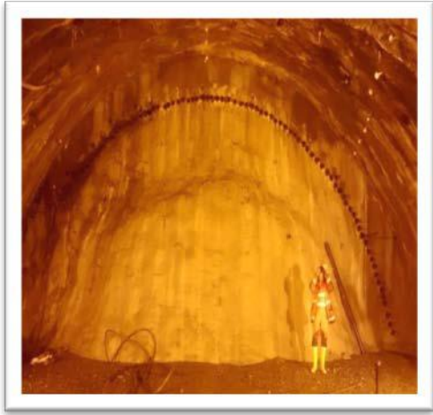
Figure 20 - Single row pipe roof
