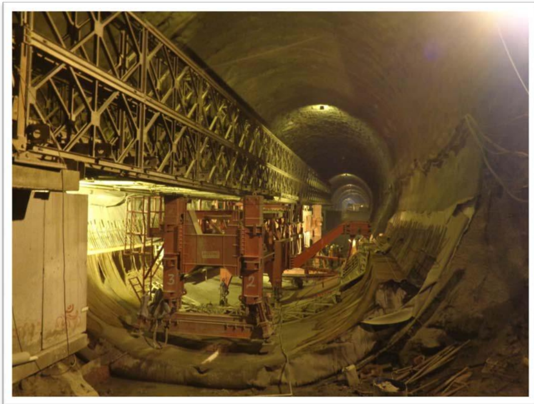
Figure 29 -Bailey bridge used for logistics in Seri Nalla zone
