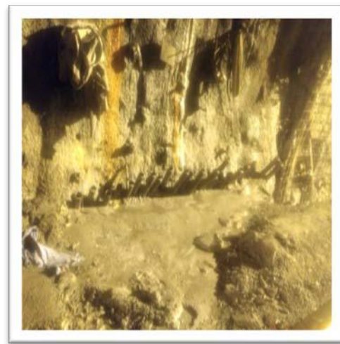
Figure- 19 Micro piling at LG base
