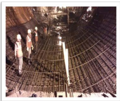
Figure 33 - Reinforcement for deep invert
