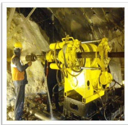
Figure 15 - Core drilling
