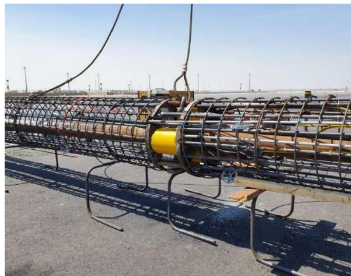
Figure 1 - BDSLT pile installation
