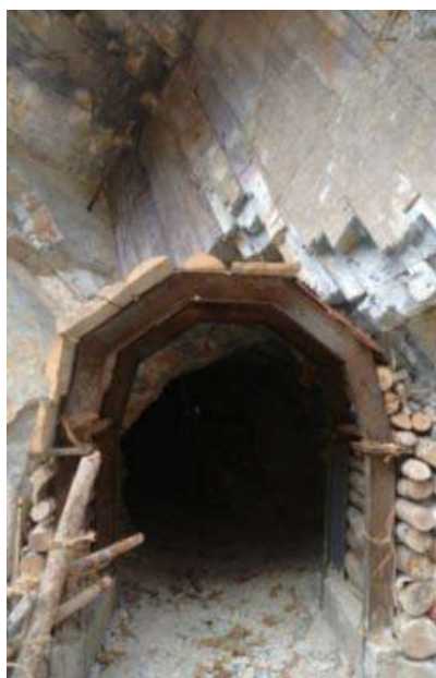
Fig. 1 - Jointing at portal of left bank drift
