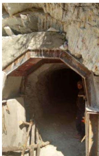
Fig. 2 - Jointing at portal of right bank drift
