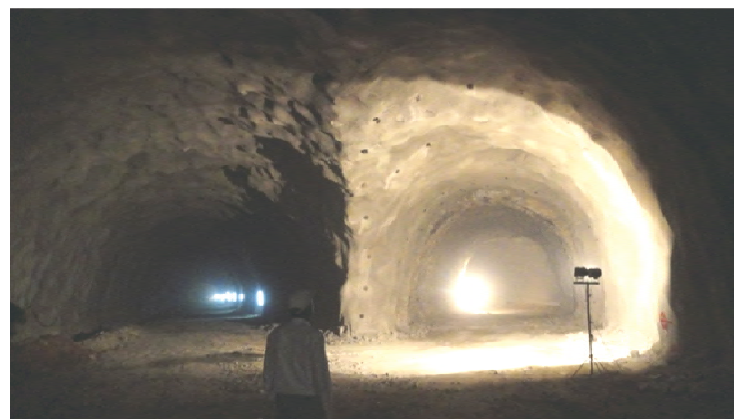
Figure 4 -Interconnecting cross passage during construction
