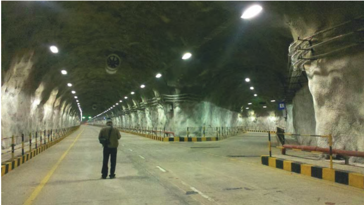
Figure 13 - Finished tunnel under operation
