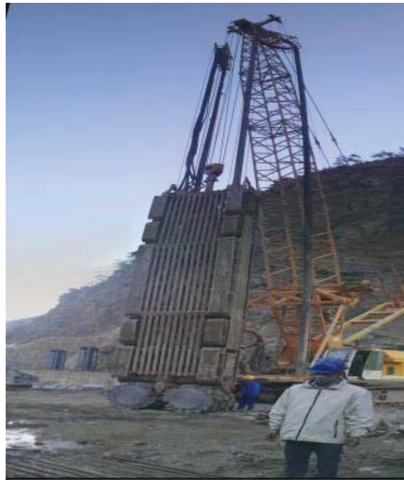
Fig. 6 - Crane mounted BC-40 trench cutter
