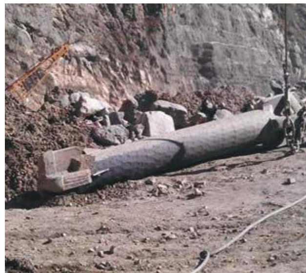
Fig. 8 - Chisel unmounted from crane unit
