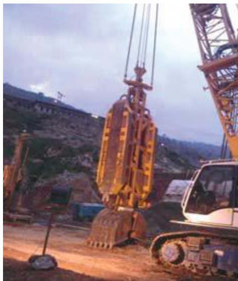
Fig. 7 - Crane mounted grab cutter
