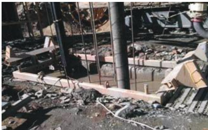
Fig. 18 - Panel immersed in bentonite
