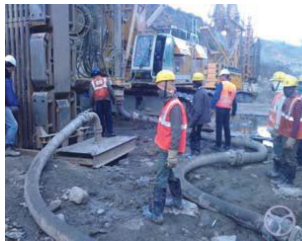
Fig. 22 - Feeder and return pipes connected to trench cutter for bentonite circulation
