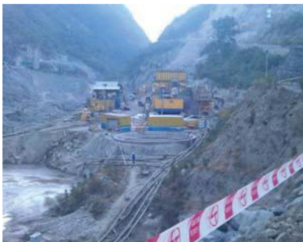
Fig. 21 - Pipe network for bentonite circulation
