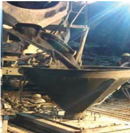
Fig. 27 - Concreting of panel
