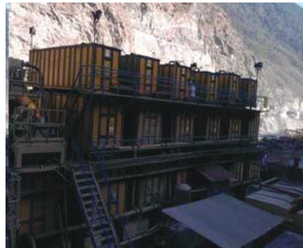
Fig. 17 - Bentonite mixing containers
