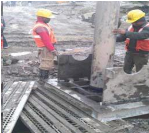
Fig. 29 - Tremie pipes being inserted for concreting of panel
