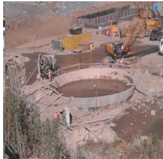
Fig. 30 - Wastebin for dumping waste bentonite at site
