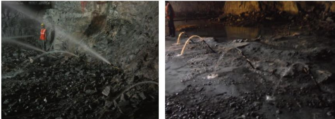
Fig. 4 - Pre-grouting for TD1 (left), post grouting for TD1 (right)
