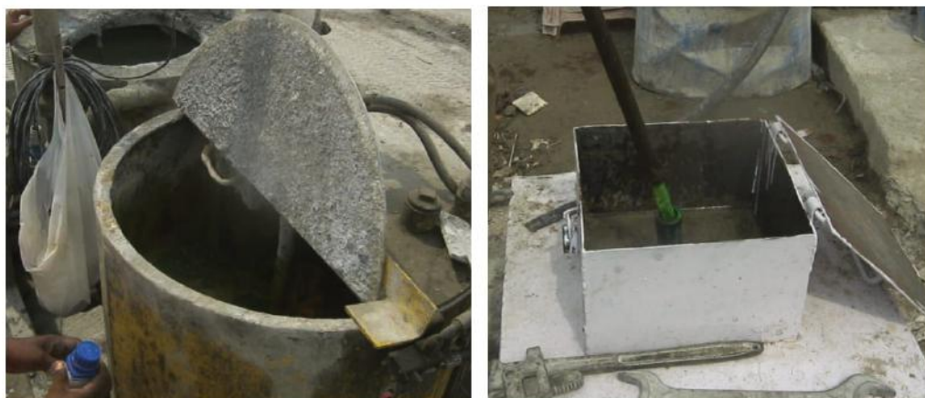
Fig. 7 - Mixing and injection of tracer material into surface monitoring borehole BH1
