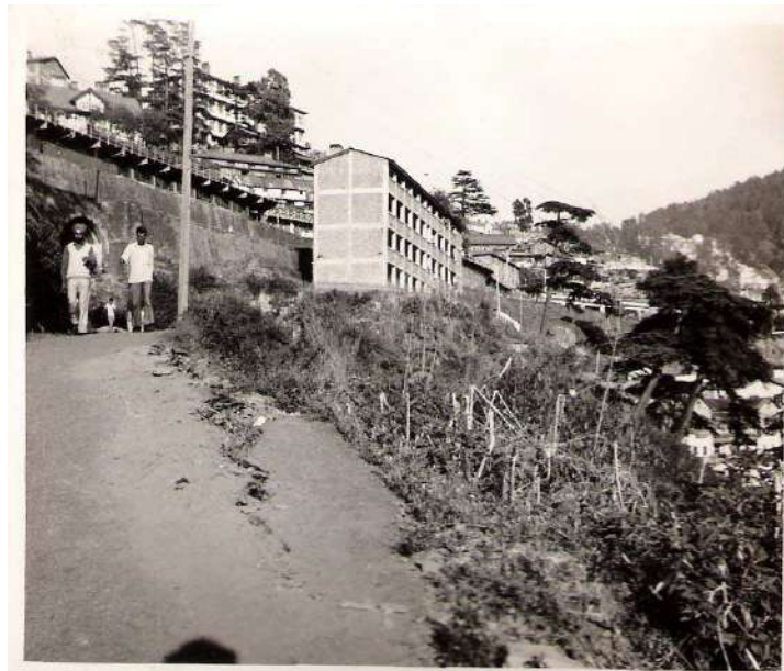
Fig. 3 - Road breaching on the way of railway colony
