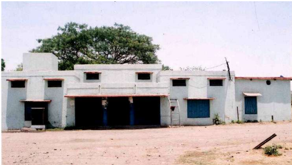
Fig. 11 – Existing structure selected for damage studies at Kamptee OCP
