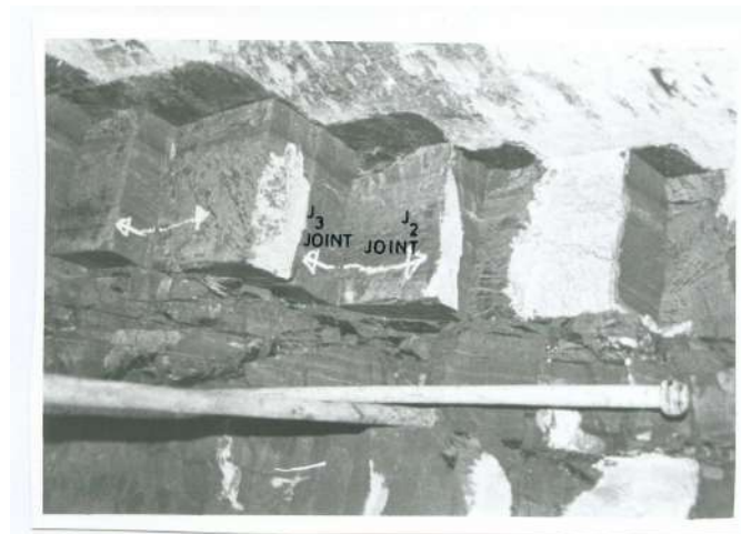
Fig. 5 – Intersection of J 2 and J 3 joints at right angle
