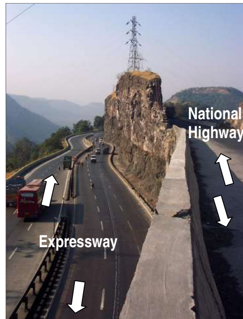
Fig. 2 – A view of Amritanjan bridge rockfall site
