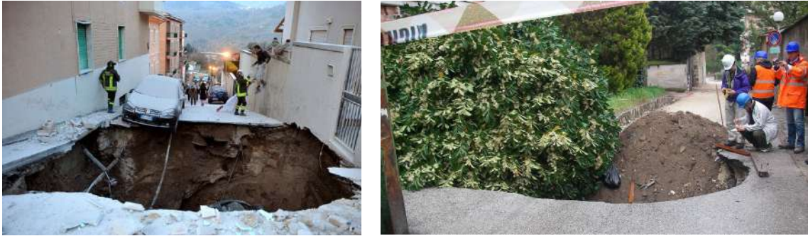
Fig. 25 - Sinkholes in L'Aquila (from Aydan et al. 2010)
