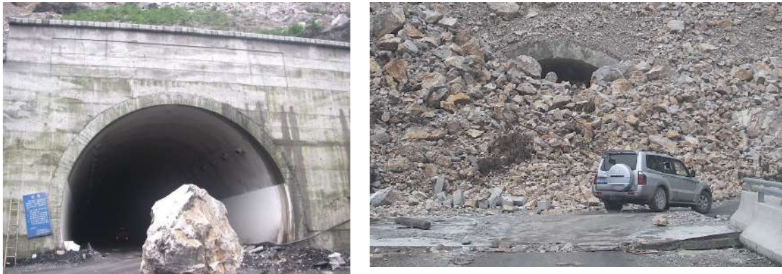
Fig. 21 - Damage to tunnel portals
