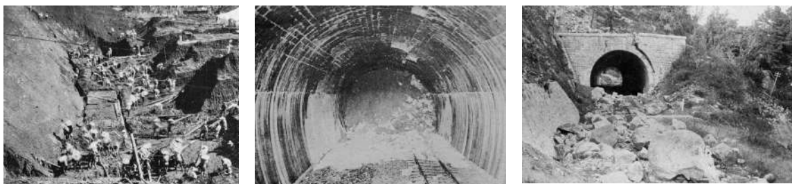
(a) Yose Tunnel
