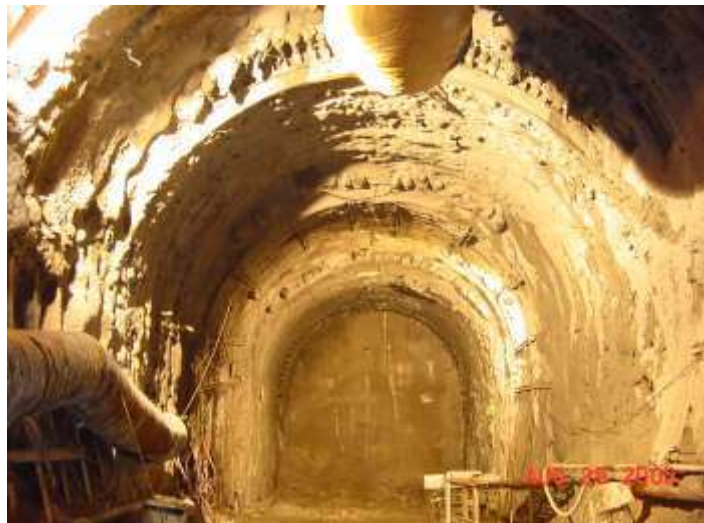
Fig. 3 - View of excavation and supporting sequence under forepole umbrella
