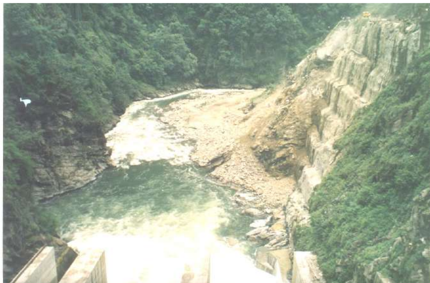
Fig. 1- Right bank slope stabilisation at downstream of the dam with PFRS
