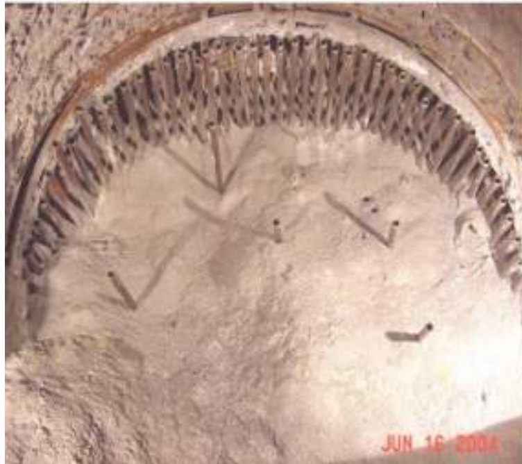
Fig. 7: Forepole umbrella with drainage holes in HRT AGO reach
