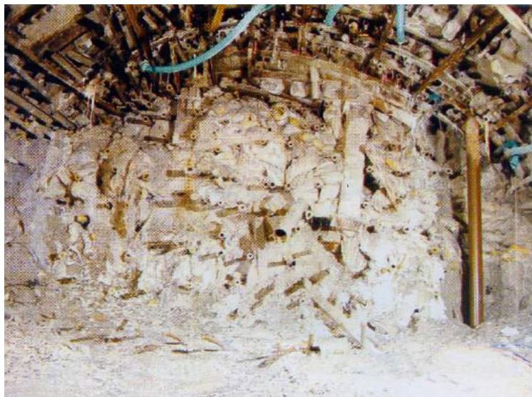
Fig. 3: Bamboo piling at HRT
