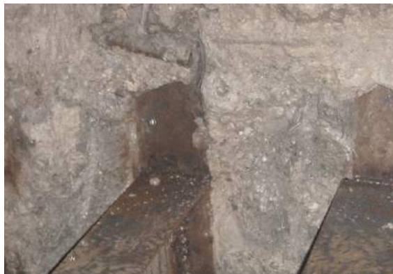
Fig. 11: Invert struts welded to the steel ribs
