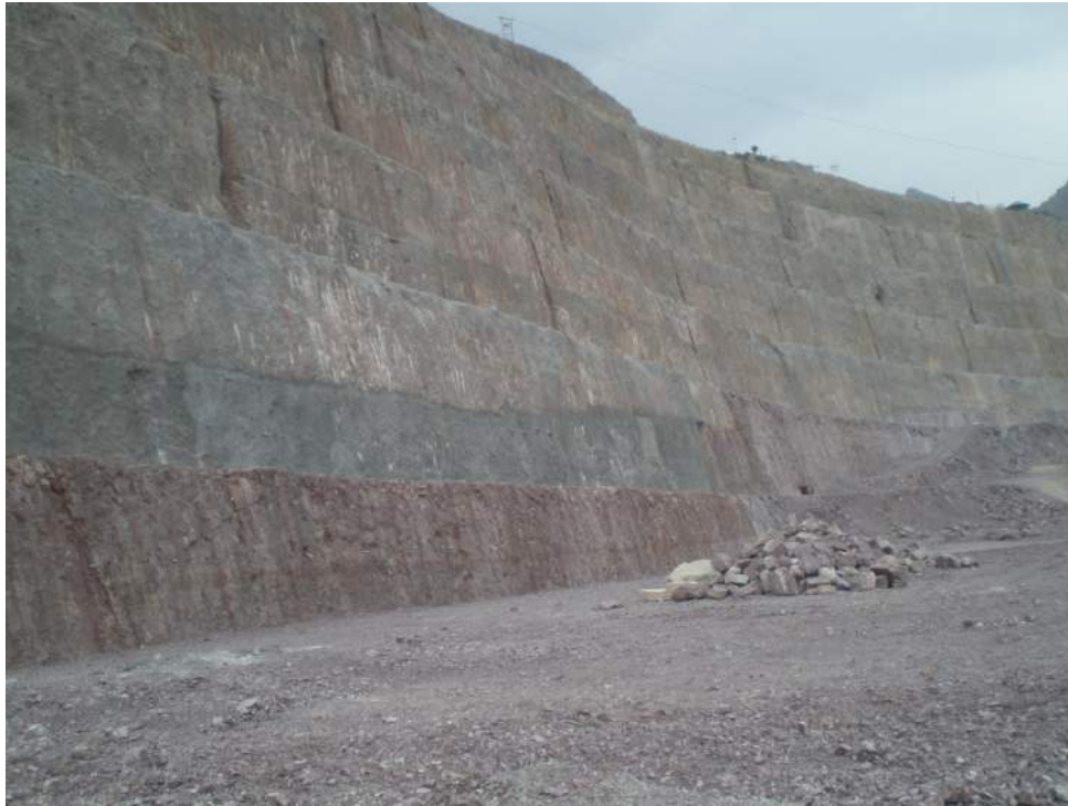
Fig. 10: Photograph showing benches of Kol dam project developed using pre-split blasts
