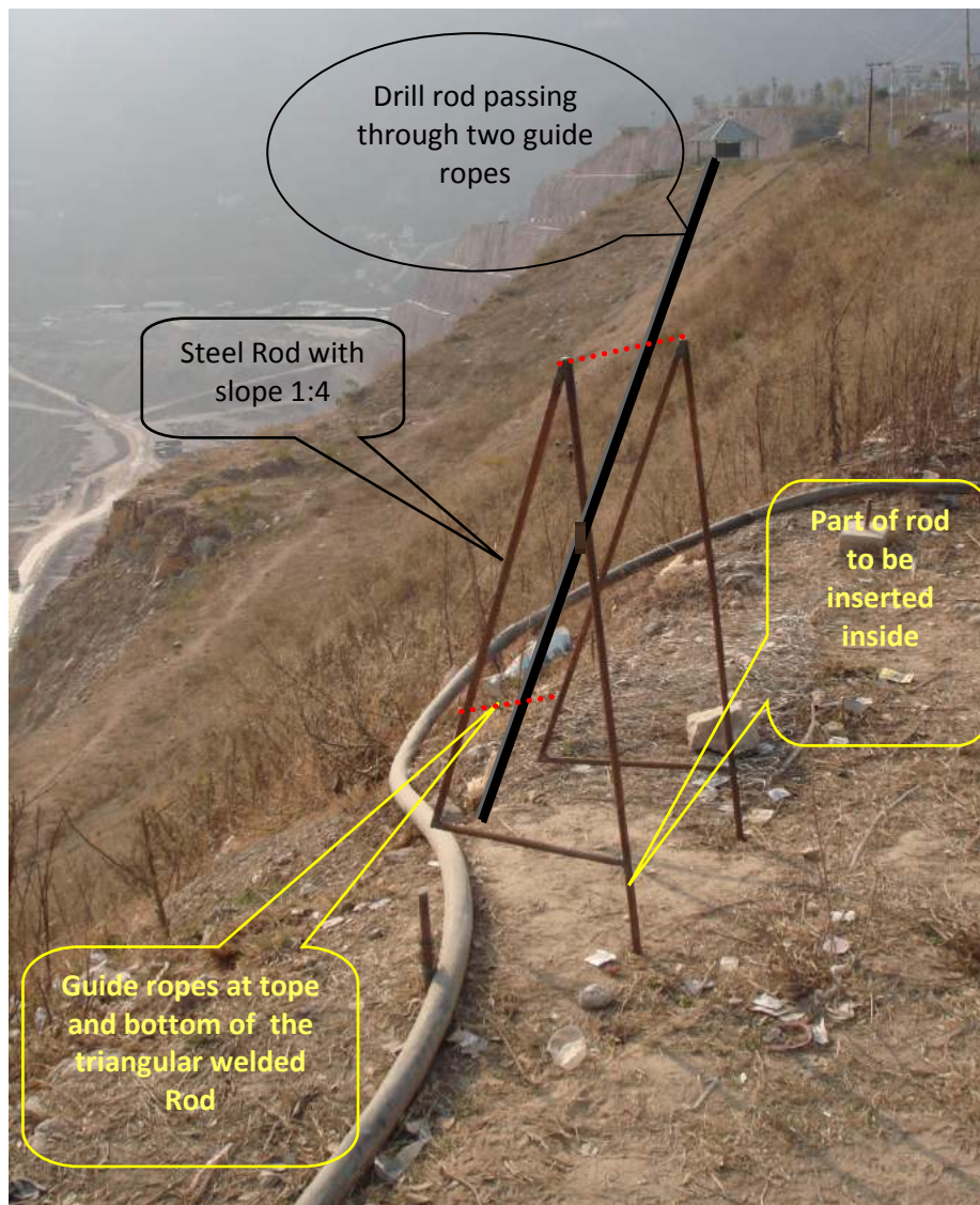
Fig. 3: Photograph showing arrangement for improving drilling accuracy at Kol dam site
