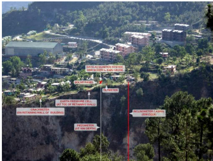
Fig. 4 - A view of instrumented landslide site from Rampur side hill
