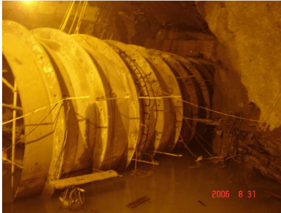
Fig. 3 - Steel liners in position
