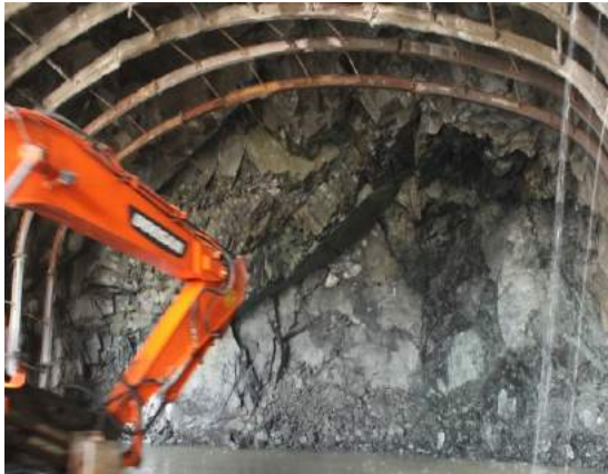
Fig. 8a - Steel rib installation
