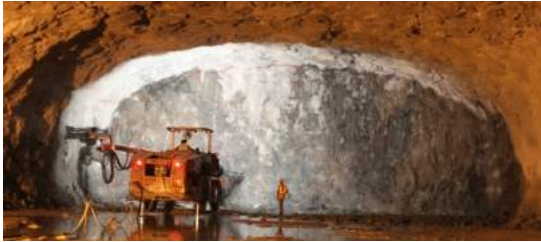
Fig. 10a - Profile marked on face before drilling
