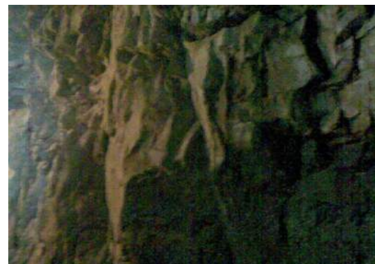
Fig. 4b - Overbreak on wall along steeply dipping shear seam
