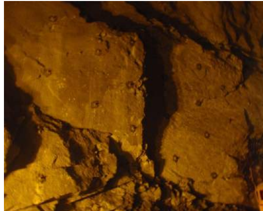
Fig. 8b - Spot bolting to prevent block failure
