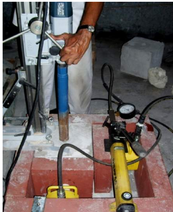
Fig. 6 - Recovery of a cylindrical core using portable core drill
