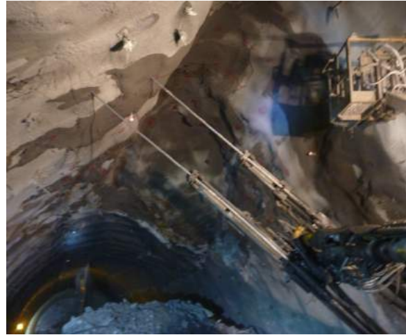
Fig.5 - Installation of extra IBO rock bolts in collapsed area
