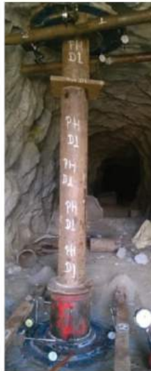
Figure 1: View of plate load test in powerhouse drift
