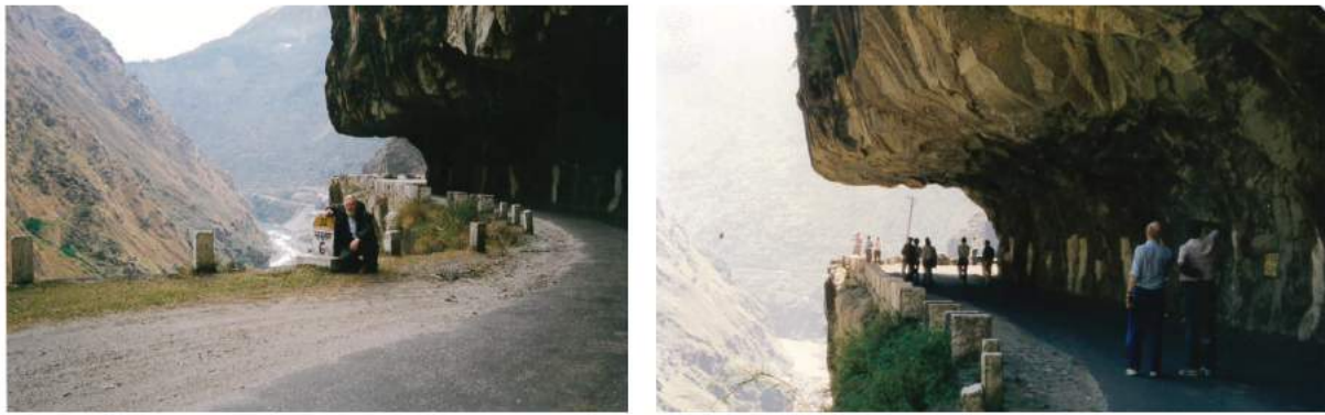
Fig. 11 - Half tunnels in Himachal Pradesh
