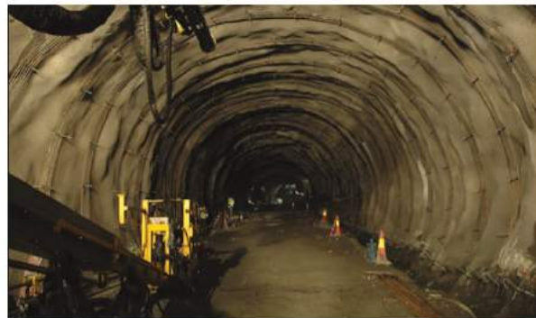
Fig. 14 - Section showing RRS and the execution of RRS in a tunnel in Oslo (Grimstad et al., 2003 and NPRA, 2010)
