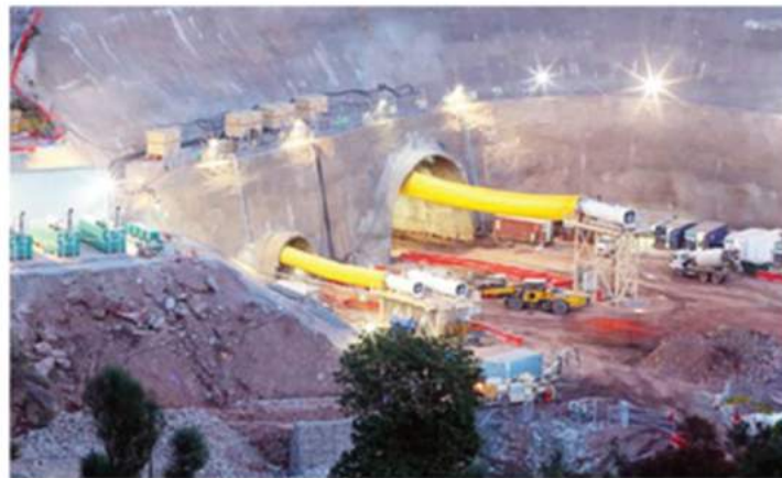
Fig. 1 - A view of Chenani-Nashri main tunnel and adjoining escape tunnel (photo: dailyexcelsior.com)
