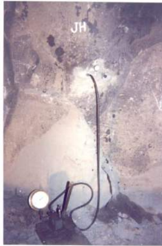
Fig.7 - Flat jack test in progress
