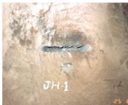
Fig. 3 - Slot cut in horizontal direction to measure vertical induced stress
