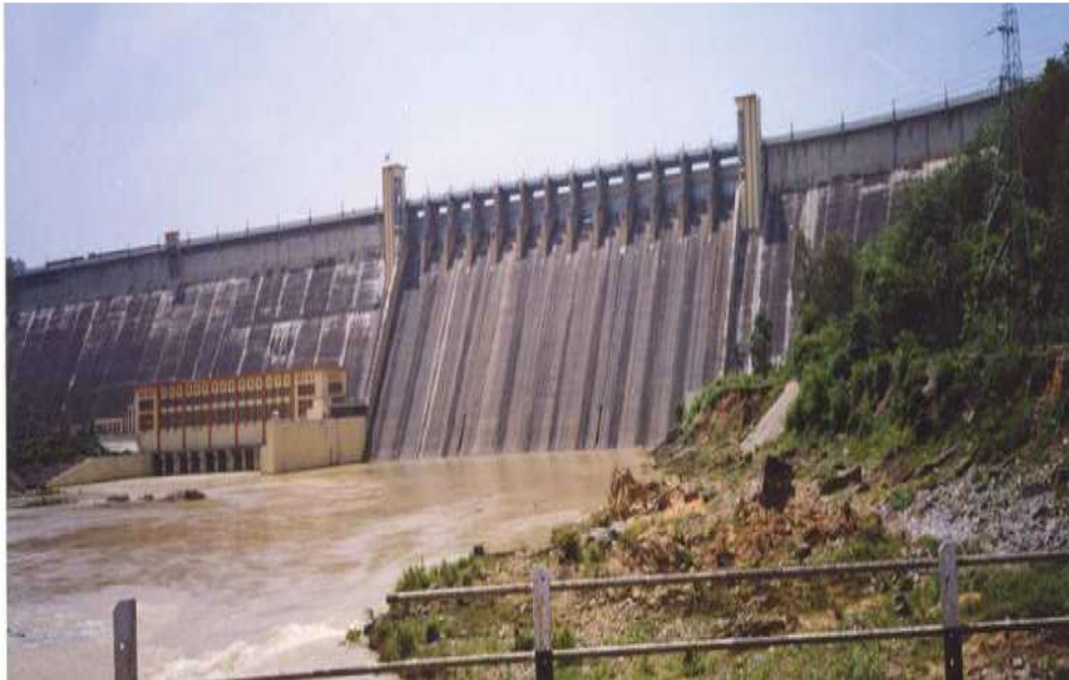
Fig. 1 - Down stream view of Rihand dam along with surface powerhouse
